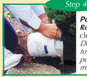
**Pour** the dry RootX down the clean out valve. Do <u>not</u> add water to the bucket, just pour in the dry mixture.
