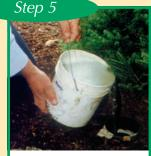
**Pour** three to five gallons of water down the clean-out after the *RootX*. You should observe some foaming in the pipe.
